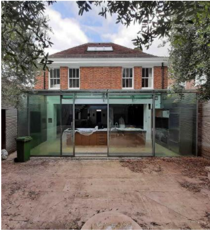
Photograph of the rear of the property
